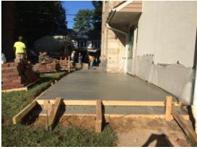
Concrete being poured for the Academy sidewalk
