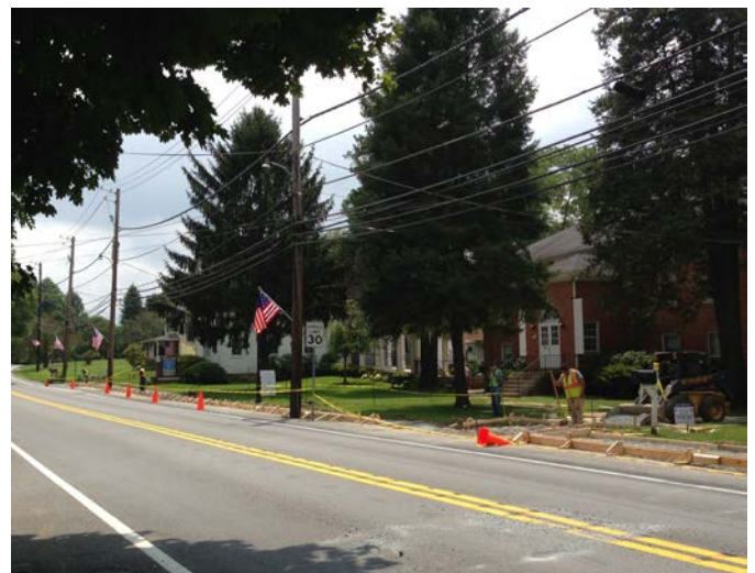
Sidewalk repairs at SUMC.
