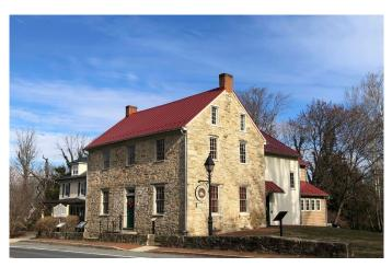
The metal roof replaces the cedar shingle roof that was installed in 1996 when the Academy went underwent a significant renovation. The installation of new gutters, downspouts, and snow guards was a part of the roof replacement project.
