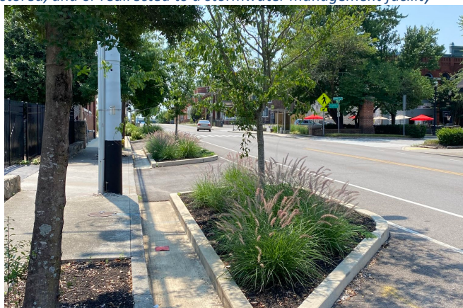
Figure 40 - Vegetated buffer strips can store and filter stormwater
